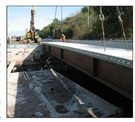
Branch of Newton Creek. Despite the project challenges, the use of ABC technologies allowed for the superstructure replacements to be successfully completed within the required closure windows over four weekends with minimal impact to the community.
