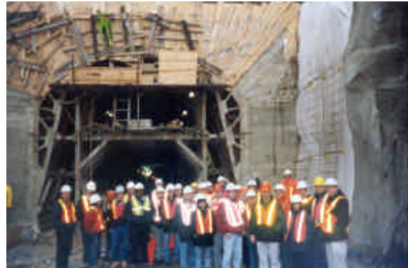
Branch members pose in front of traveling formwork specially designed for the Bergen Tunnel Project
